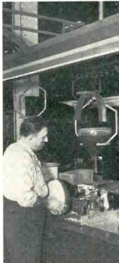
FIG. 4—Overhead tube conveyor dips down at end of each main assembly line to make picture tubes available exactly where needed. Conveyor also brings tube clamping strip
