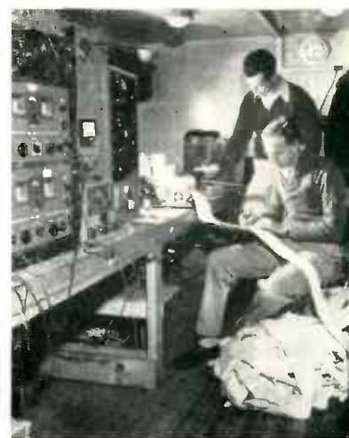
Continuous-wave meteor recording apparatus permits study of swarms of meteors too small for photographic recording
